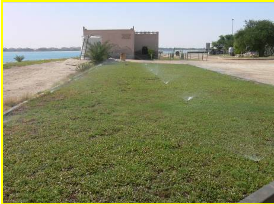
Fresh water top-surface irrigation system. (Conventional)
