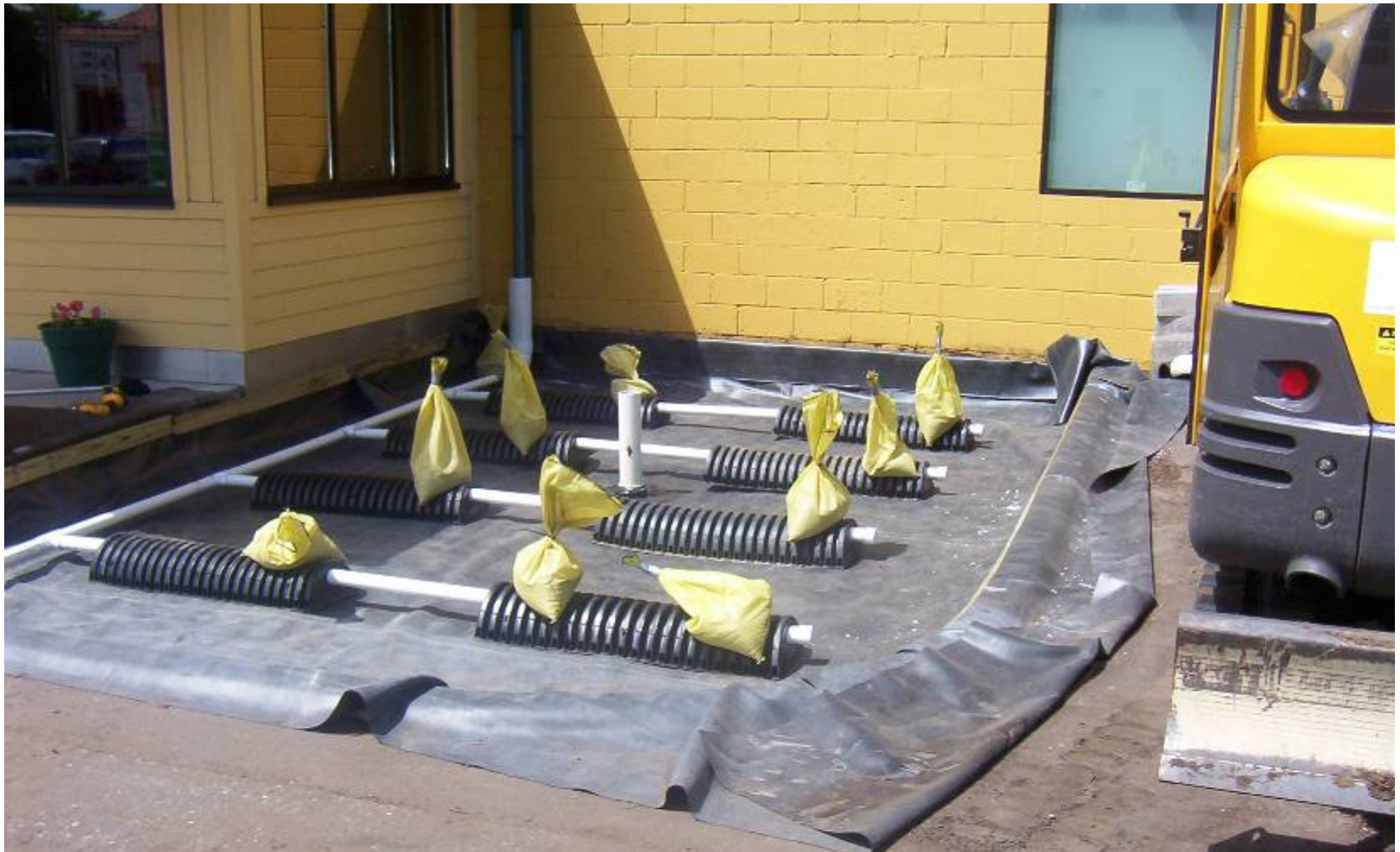
Liner, Chambers and Pipes
