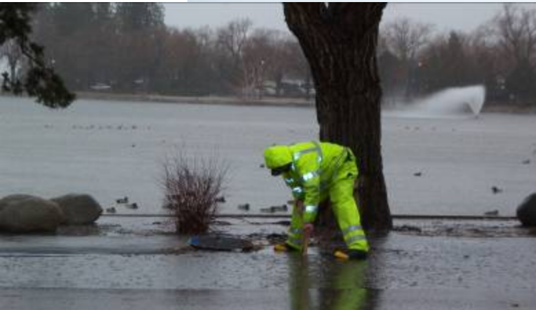
City Maintenance works during storm to unclog storm drain.
